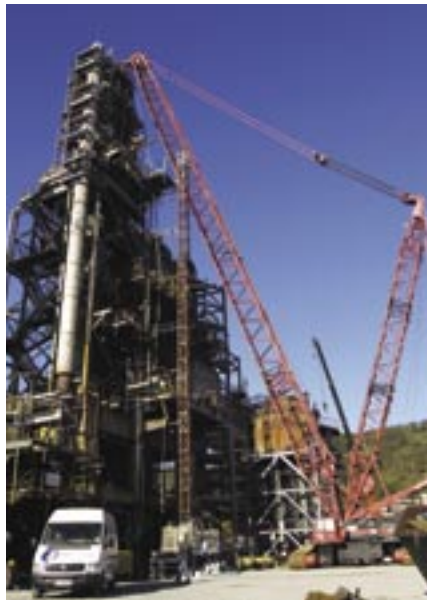
A 450-tonne 'American' crane prepares to lift a platform up to the regenerator of the cat cracker during shutdown.
